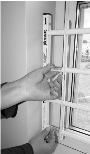
Step 1 Locate all emergency release buttons indicated by labels.
